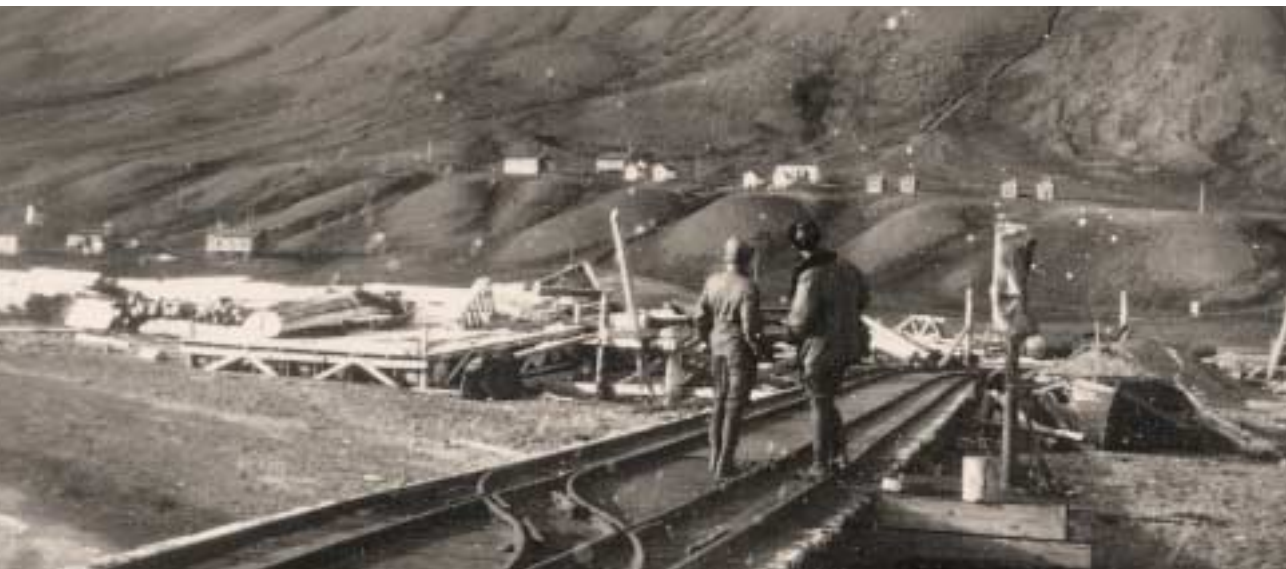
The Hiorthhamn facility seen from the quay mid 1920s.
