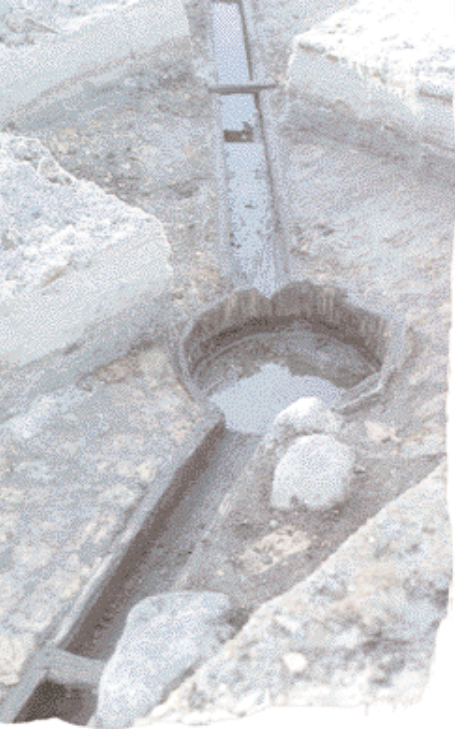
A complex system of drainage gullies carried away the surface water so that one was able to walk dryshod along the cobbled alleys of Smeerenburg. Exposed during the excavations at Smeerenburg in 1979-80.
