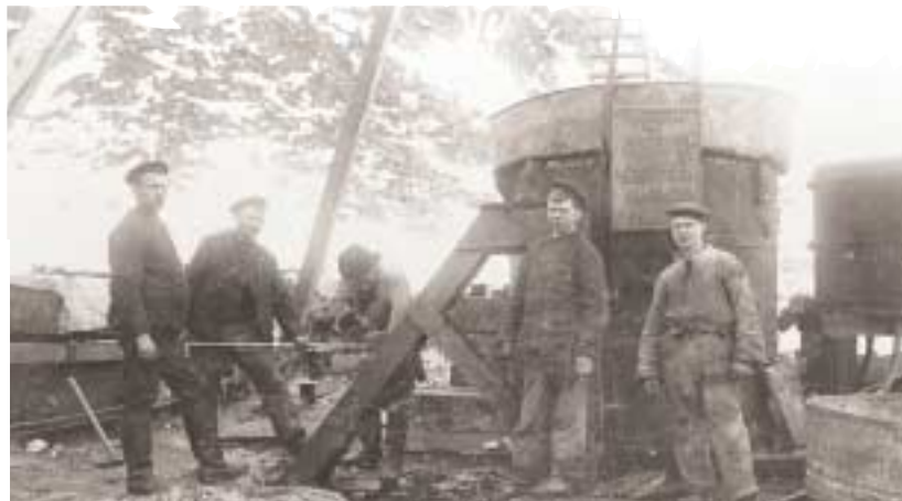
The expedition crew built a gas plant that produced 5000 m 3 hydrogen from 2-3 tonnes of iron filings, 41 tonnes of sulphuric acid and 76 tonnes of salt water - in addition to 450,000 litres of rinsing water. Above we still see remnants of the felt that protected the Eagle inside the balloon hangar.
